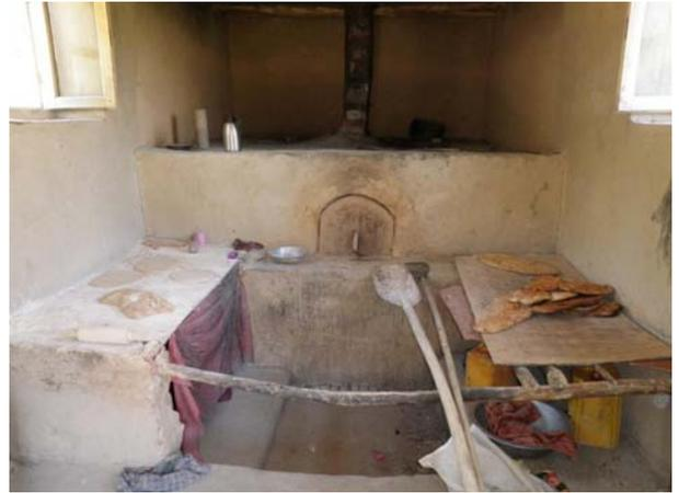
New energy efficient stove: coal is used as fuel, fire is set in a separate chamber which is accessed only from the outside; smoke escapes via chimney out of the building. (Photo: Helvetas)
